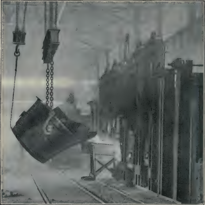
CHARGING A FURNACE WITH MOLTEN IRON FROM MIXER
